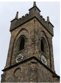
The open joints in the masonry, specifically the stone plinth remain and have not yet been fully addressed, however. There is a need to carry out some fairly urgent repointing of the open brickwork joints to the tower, so this should all be addressed in the near future under a separate programme of works.
